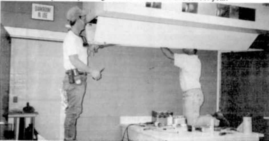
Construction workers hard at work in the art room.
