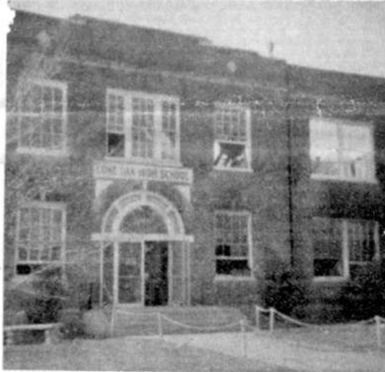
VIEW OF SCHOOL ENTRANCE showing damage to upstairs classrooms.
